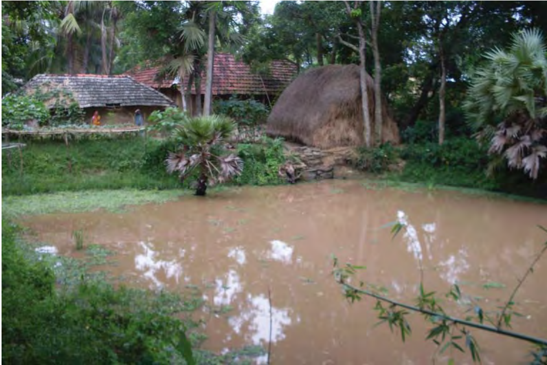
Houses in the floodplain regions of Orissa and West Bengal, built on raised mud platforms. The adjacent land, from where the mud has been excavated, forms a pond rich in SIFFS
